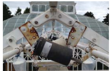
Pneumatic actuator for vent sash.
