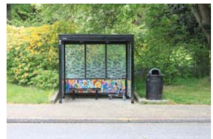
Bus stop does not indicate location.
