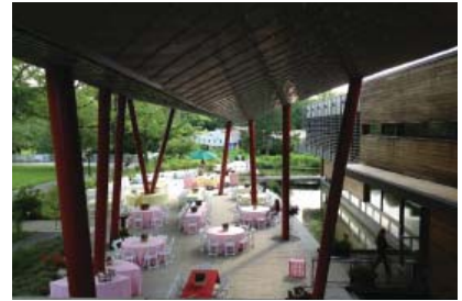
Wastewater bio-treatment pond, located adjacent to the tables.
