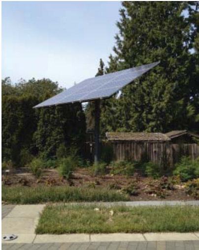
Example of solar panel structure.
