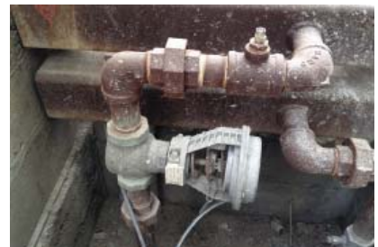
Pneumatic actuator for heating system.
