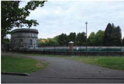
Pump house and Reservoir.
