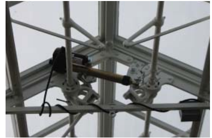
DDC controlled linear actuator.
